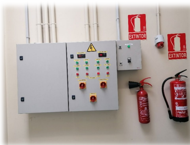
Fire extinguishers (powder and CO2) at the entrance and emergency cryptograms inside the Necropsy Room.
